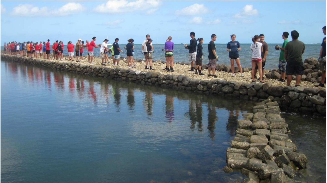
Figure 7: Wall restoration project at He'eia. Photo Credits: Paepae o He'eia
